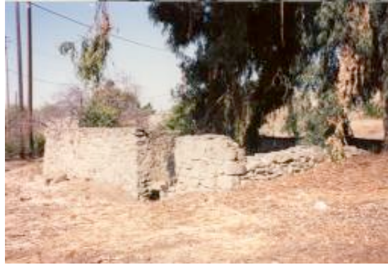
Remains of the Vallejo Flour Mill, which once served nearby Mission San Jose
