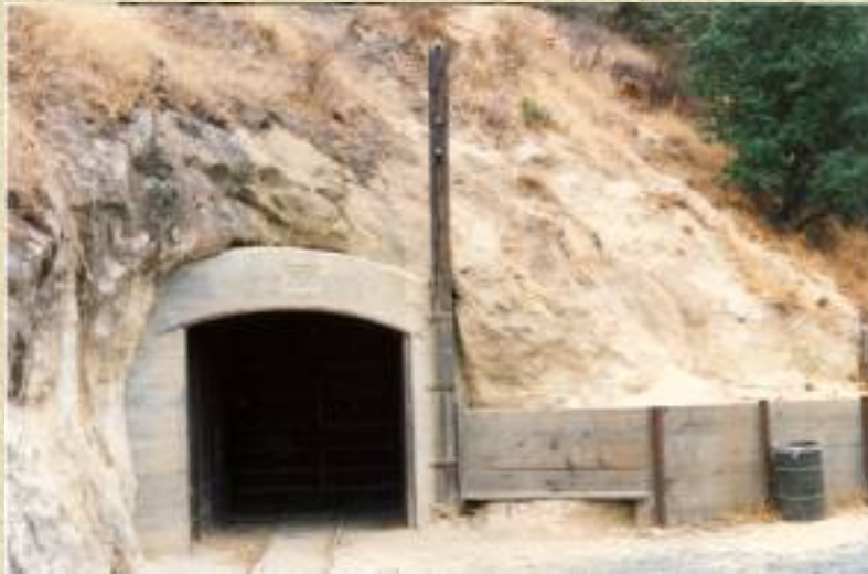
Hazel-Atlas mine portal (1930) - used for sand mining (Somersville)
