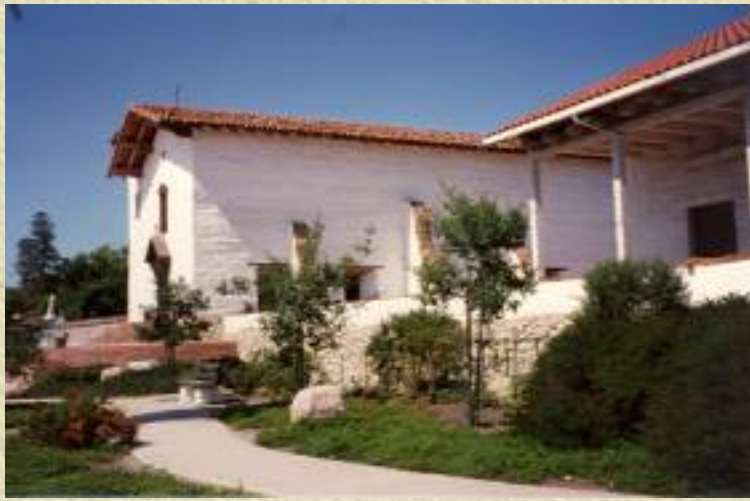
Reconstructed Mission Church. The church has walls 4-5 feet thick.
