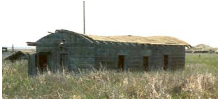
Gordon Gun Club, built in 1880. The first non-railroad structure on the island.
