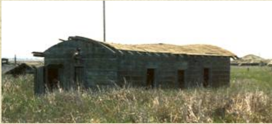
Gordon Gun Club, built in 1880. The first non-railroad structure on the island.
